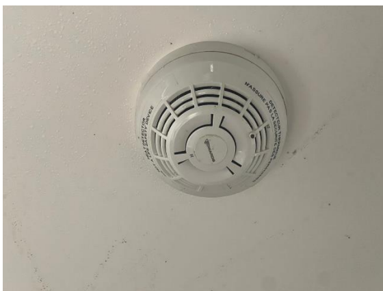
Rate of Rise Heat Detector
